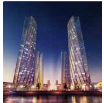
Lusail Plaza Towers - Qatar
